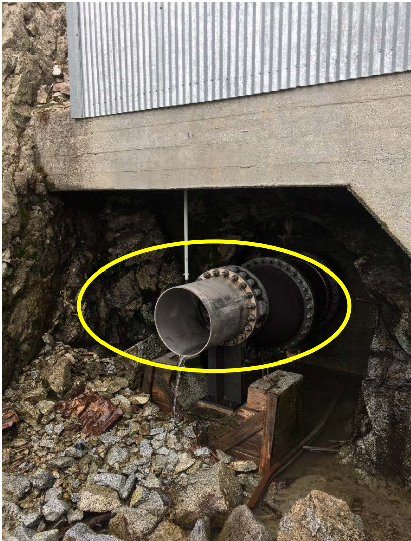
Figure 2-4. Existing butterfly valve and valve support (circled in yellow).
