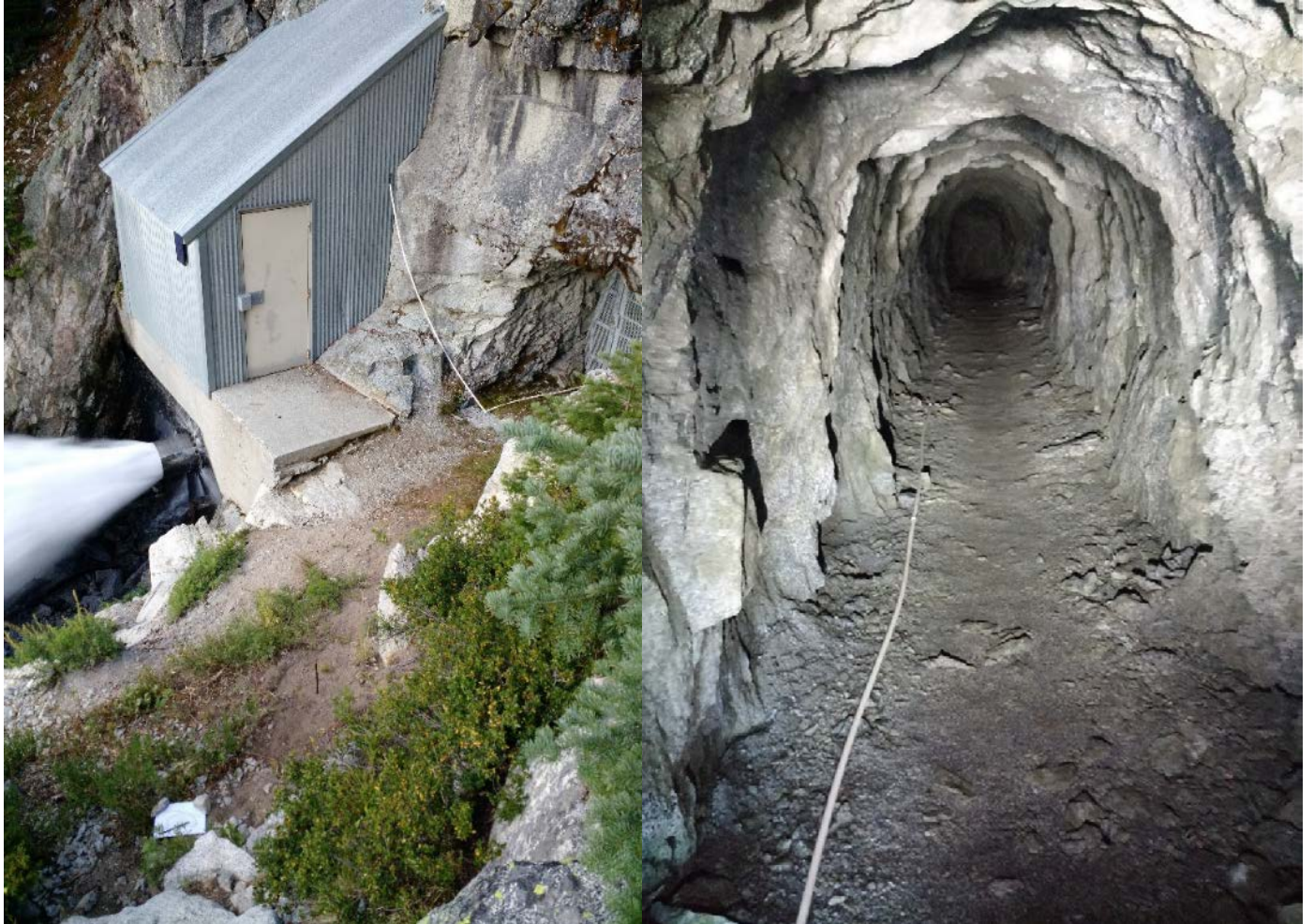
Figure 2-3. Adit Tunnel entrance located to the right of the valve control house (shown at right in left photograph) and Adit Tunnel interior (in right photograph).
