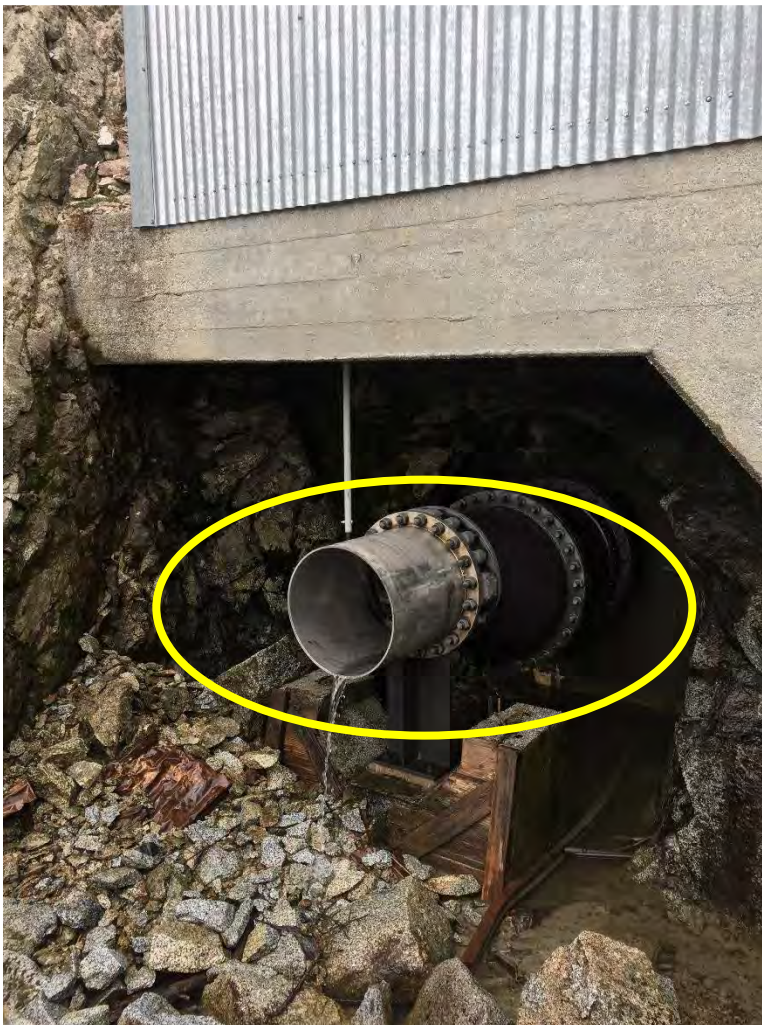
Figure 2-1. Existing butterfly valve and valve support (circled in yellow).
