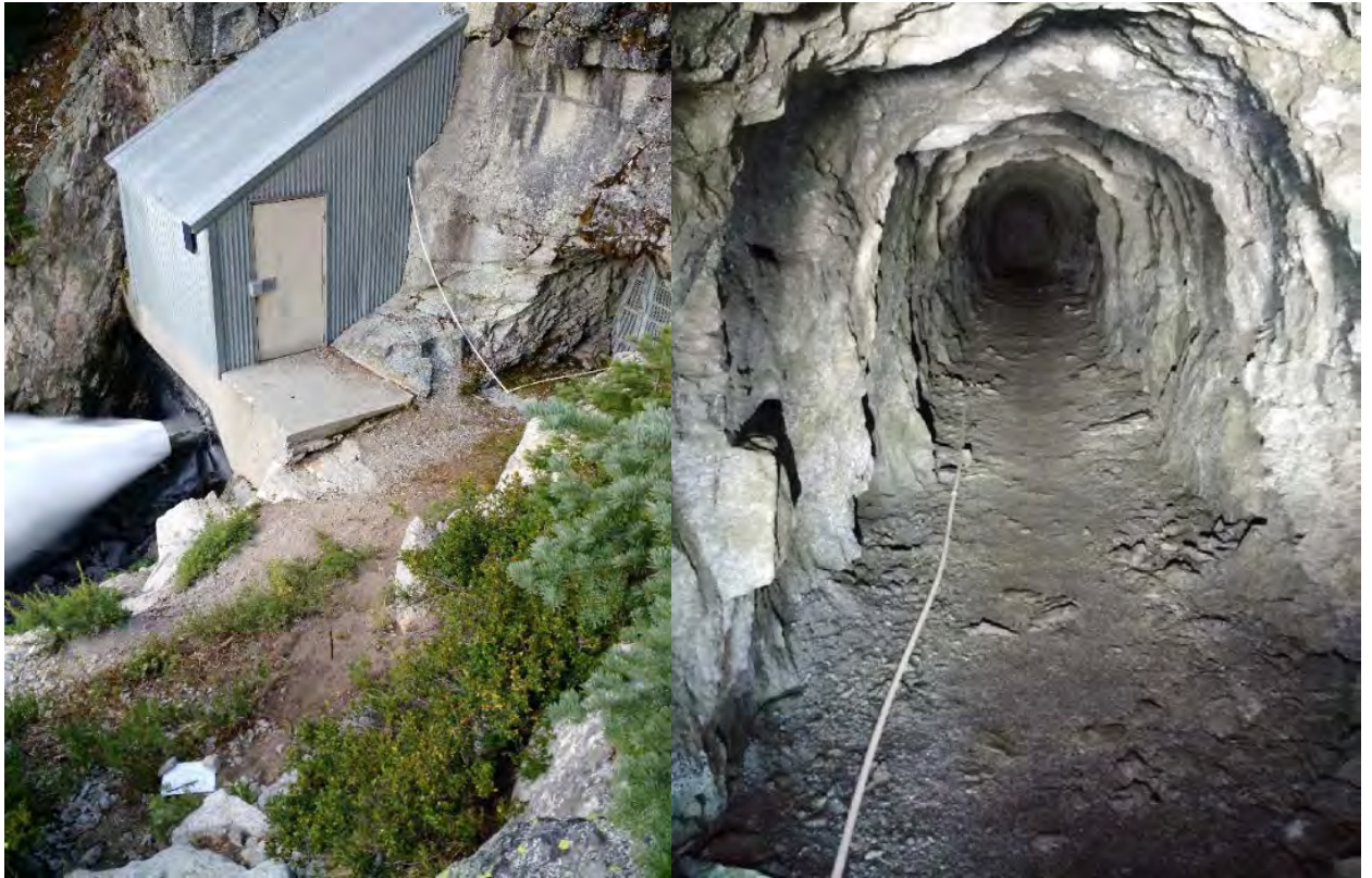
Figure 2-3. Adit Tunnel entrance located to the right of the valve control house (shown at right in left photograph) and Adit Tunnel interior (in right photograph).
