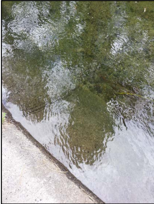
IPID Ditch – partial lining
