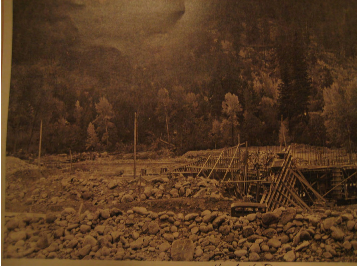
(Figure 10) This photo shows Dam 2 (also referred to as the Headgate Dam) under construction in 1938. This photo shows the type of material underlying this area of the Leavenworth Valley. It is obvious that the underlying material is composed of small boulders that appear to be water worn. It is not hard to imagine that this area is a place of aquifer recharge. Compare this to Figure 4, on page 5, a photo of approximately the same area in 1929 (that photo was taken from a position slightly upstream and to the left of this one)
