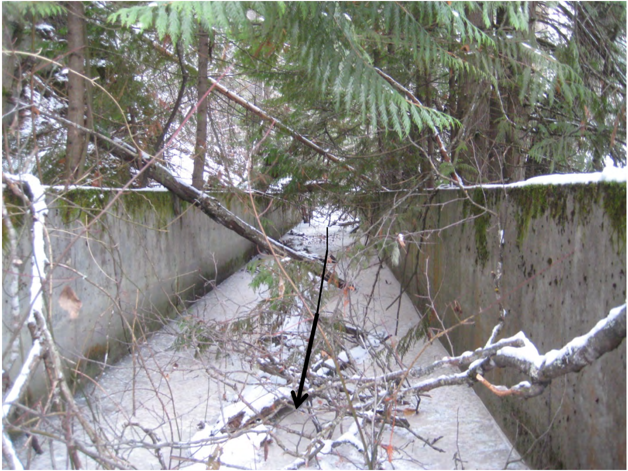
(Figure 15) This is another photo taken in 2013 of what is left of the Wenatchee Canal. The canal was abandoned within a few years after operating because Wenatchee River water was too warm and the plan to pump Wenatchee water to the Icicle Irrigation canal failed.
