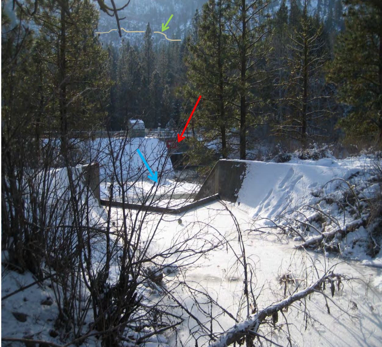
(Figure 16) This photo, taken in 2013, shows the southeastern end of the Wenatchee Canal. The plan was to discharge Wenatchee River water into the southern end of the Hatchery Canal shown here in the center of the photo, where it would flow through Dam 2 (Headgate Dam) to the pools holding anadromous fish until they were ready to spawn. The Headgate dam is across the Hatchery Canal in this photo. (A red arrow points to it).
