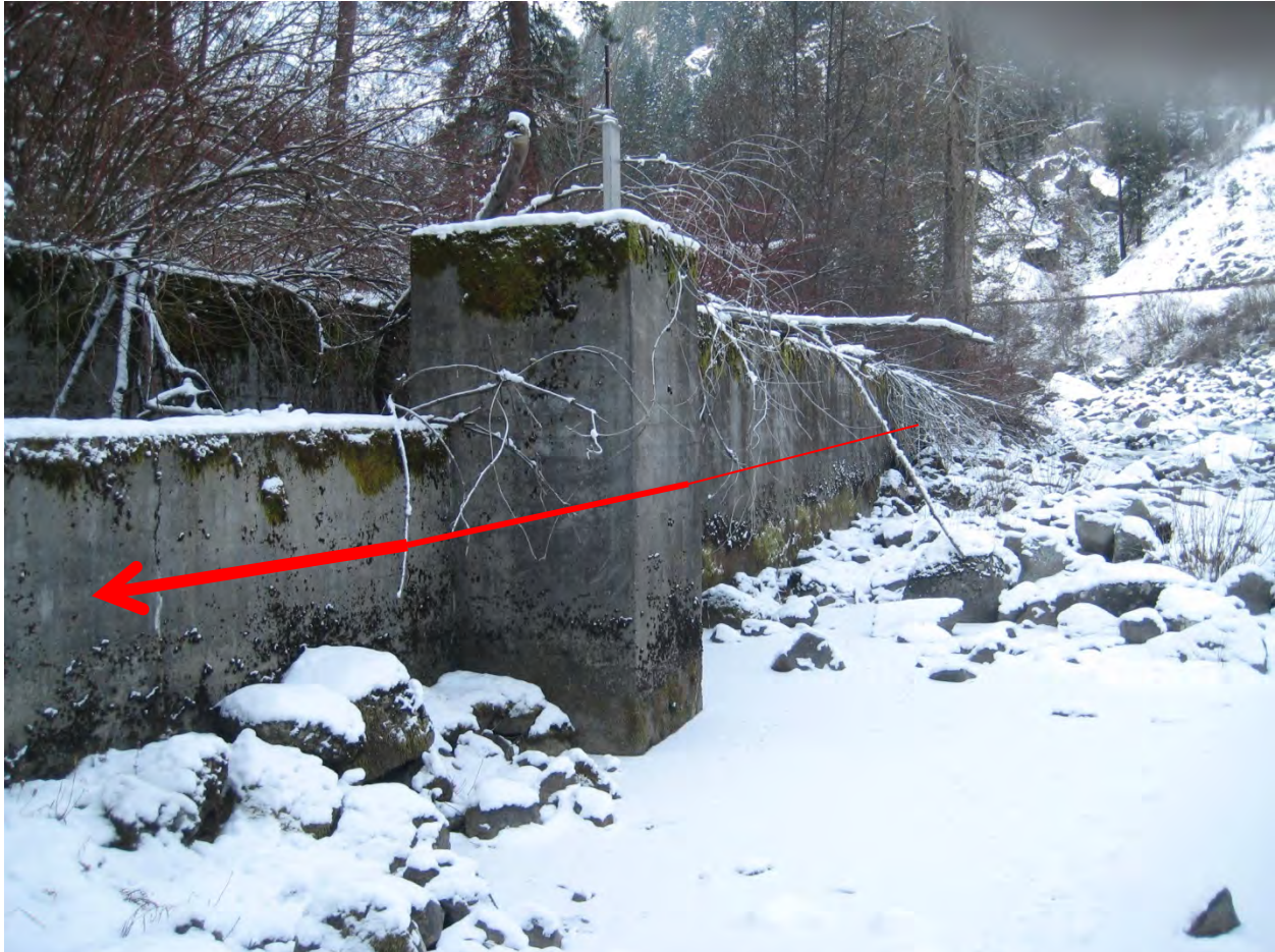
(Figure 14) This is a photo taken in 2013 of the Wenatchee River Canal. This shows the canal as it leaves the Wenatchee River in Tumwater Canyon. A large steel drum gate is mounted in this section of the canal to control water volume at this point in the canal. The red arrow shows direction of water flowed.
