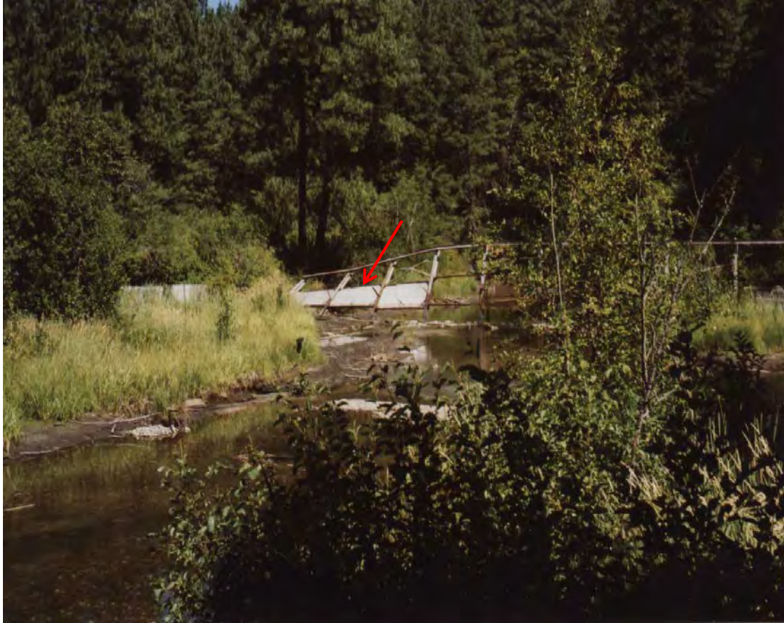
(Figure 20) This is a photo taken in 2001 from the walkway on Diffusion Dam 4 looking downstream. The rack was damaged by the 1990 flood (red arrow).
