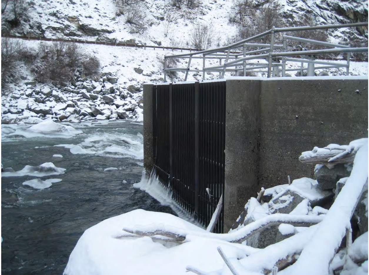
(Figure 13) This photo shows the headworks of the Wenatchee Canal. The photo was taken in the winter of 2013. The road across the river is Highway 2 in Tumwater Canyon about one mile west of Leavenworth.
