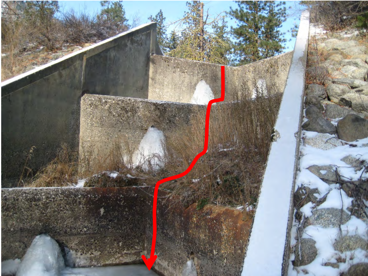
(Figure 17) This is the discharge end of the Wenatchee Canal taken in 2013. The series of steps is a design to get water from a higher elevation to a lower elevation without eroding the bottom of the canal. The red line with an arrow at the end shows how water cascaded to the floor of the Hatchery's Canal.
